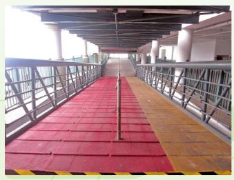
鋪有防滑物料及設有槽紋的碼頭斜道 Ramps with anti-skid gangplanks and grooves at pier
